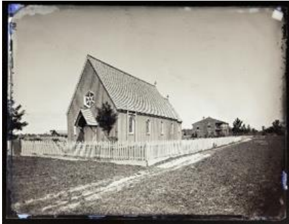
Figure 1A. St. Mark's Church Palatka. Photo by Mathew Benjamin Brady, c.1870. Photo courtesy Canadian Centre for Architecture, Montreal, Quebec.
